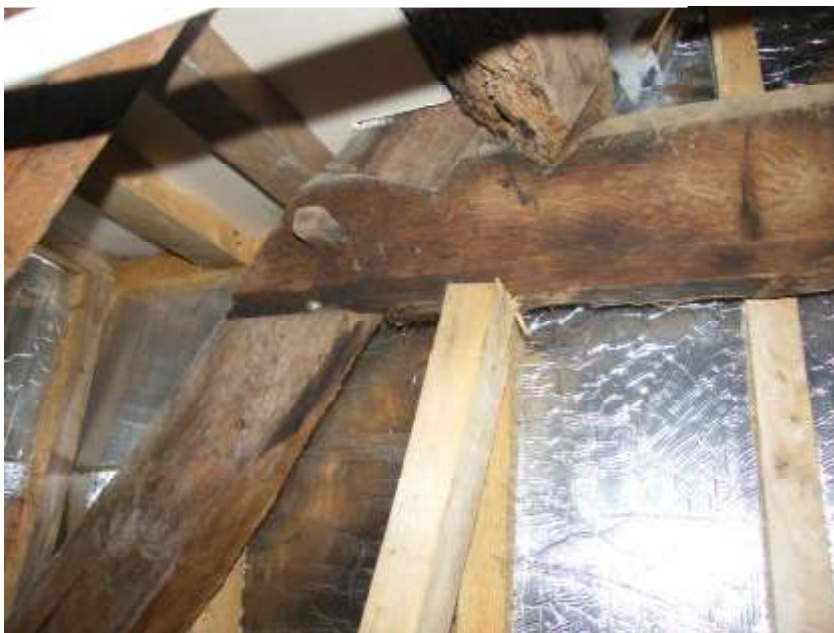
Clasped purlin truss near east gable
