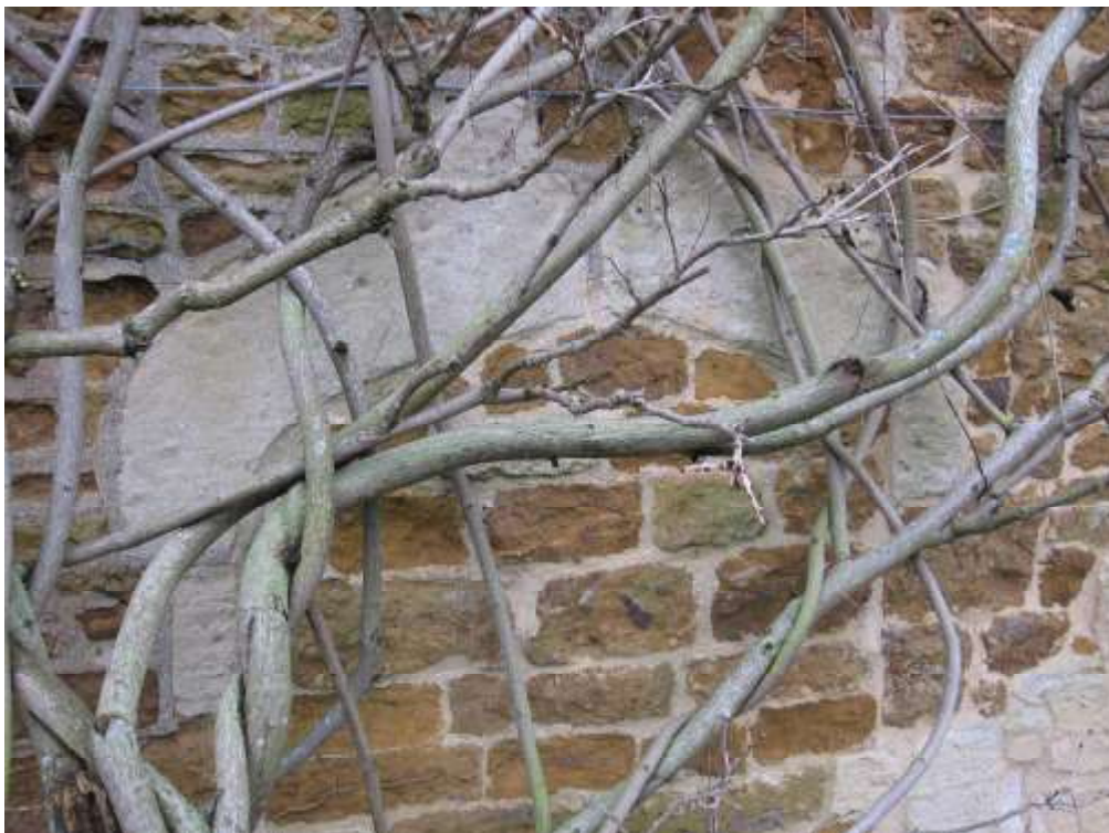
Detail of four-centred arch head to southern doorway
