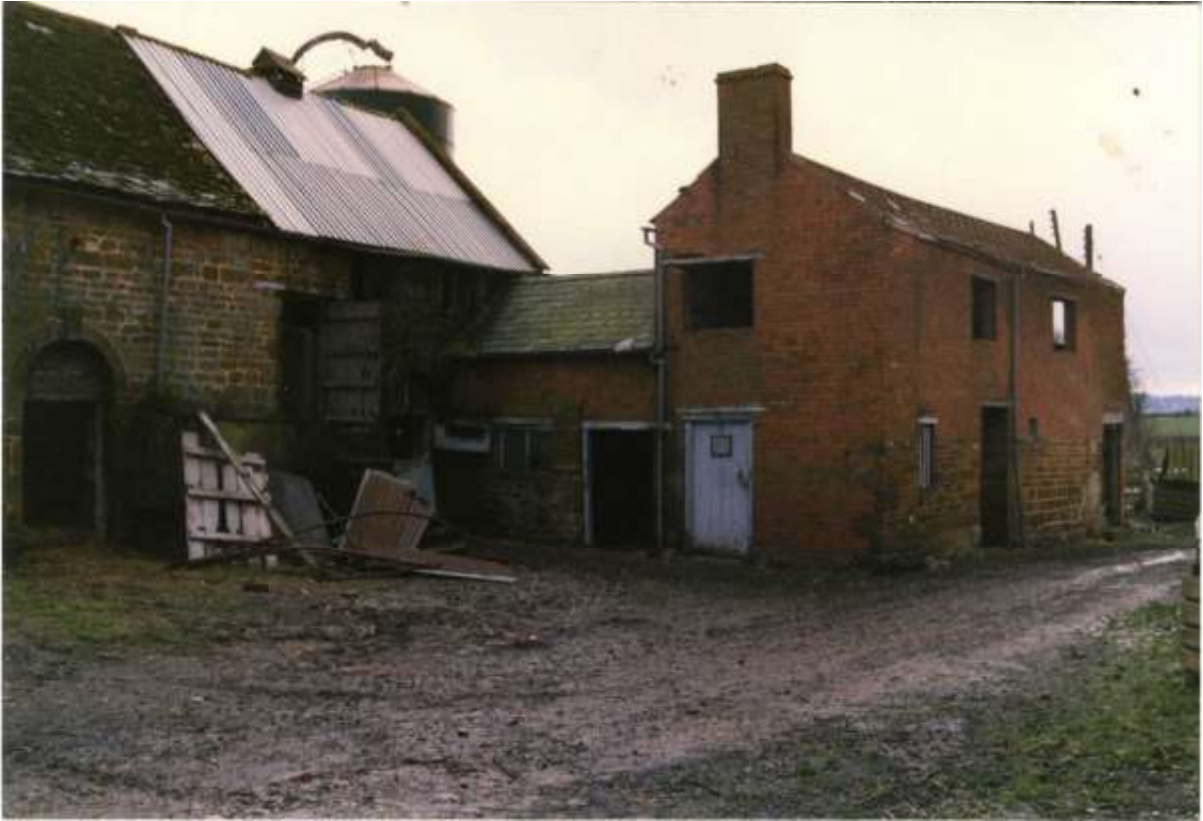
View of the barns from the north in 1987 before rebuilding
