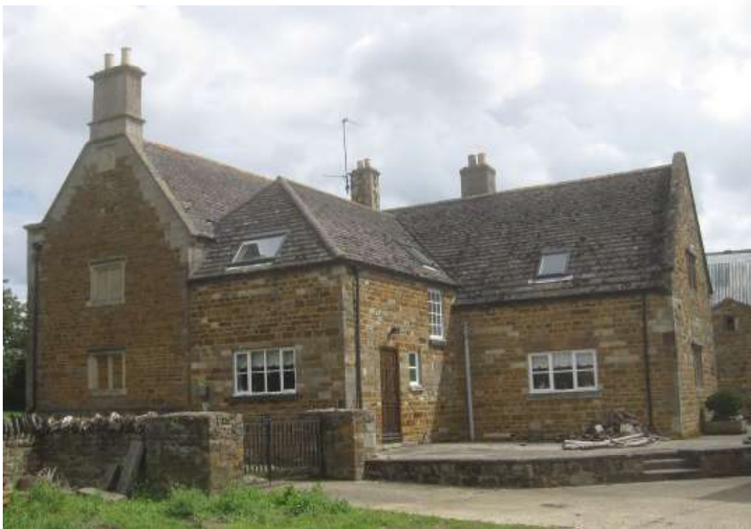
View from the north-west
