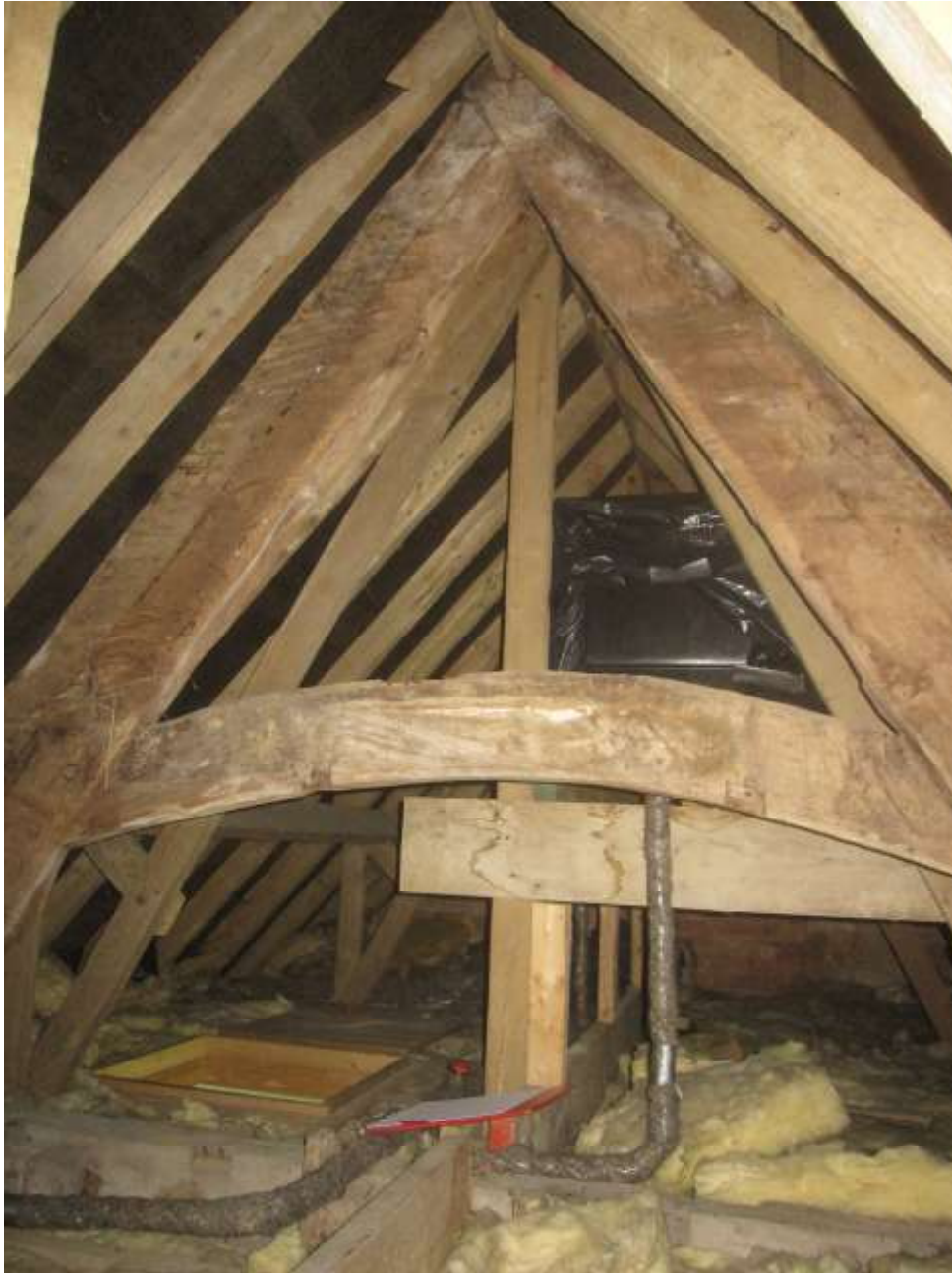
Roof truss T2 to the main range
