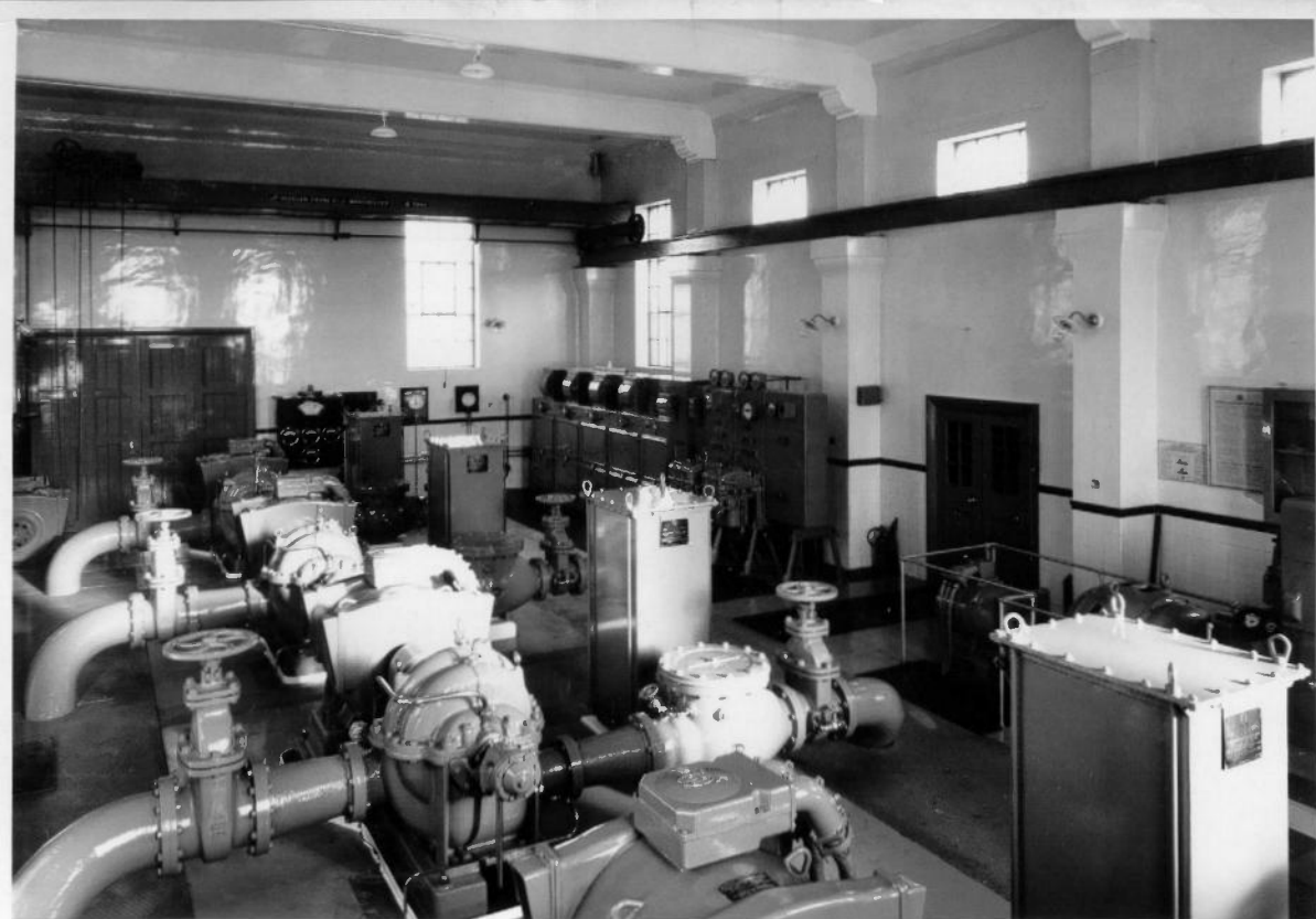
P24 Caldecott pump house
