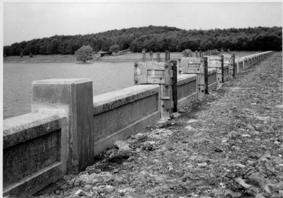
EYE BROOK DAM RAISING WAVE WALL
