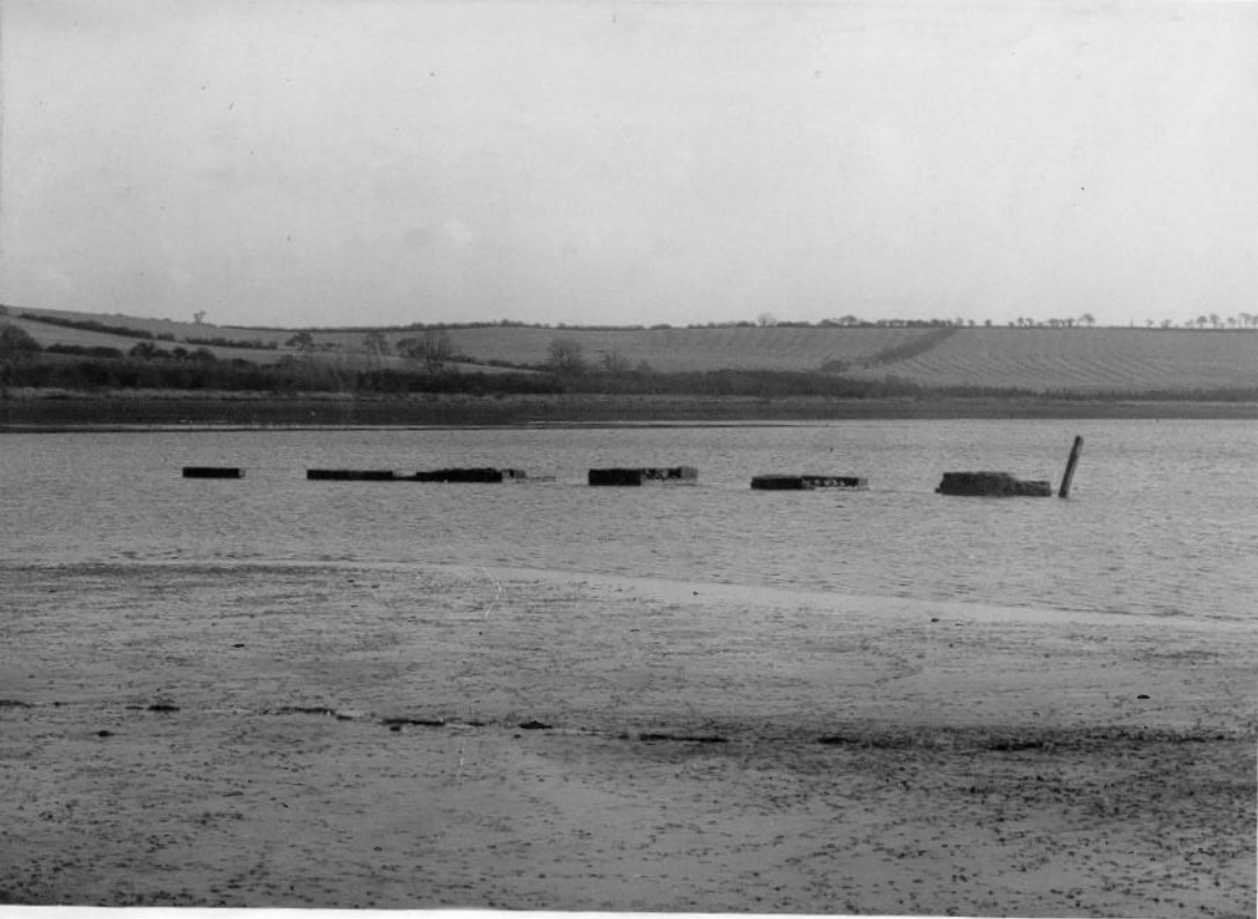
The old foot bridge at Stoke Dry, taken 20th December 1955 when the water level was 212.89 feet O.D. - over 14 feet below new top water level of 227.50 feet.
