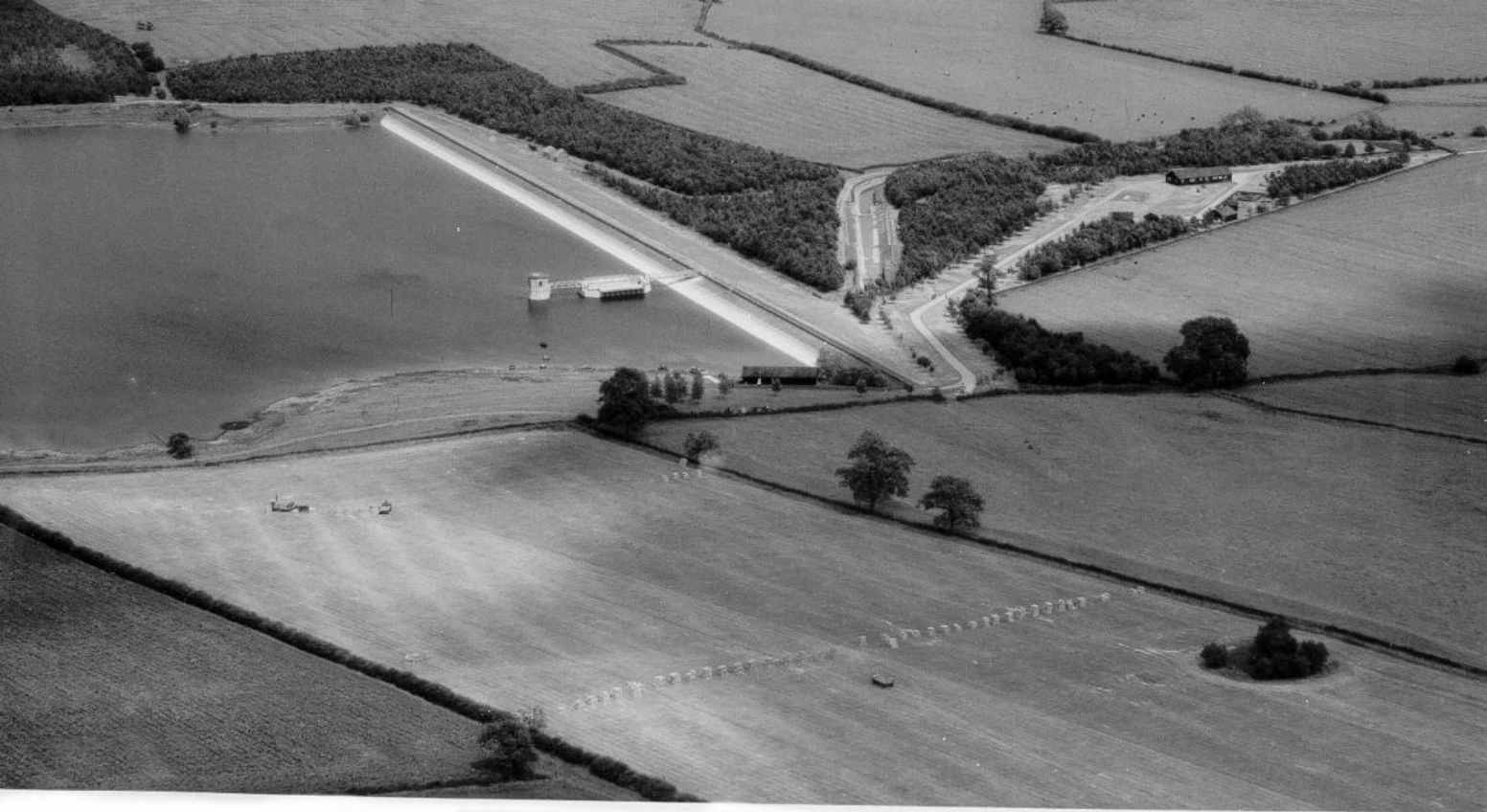
Aerial views of Eye Brook Reservoir, showing siphon spillway. June 1957.
