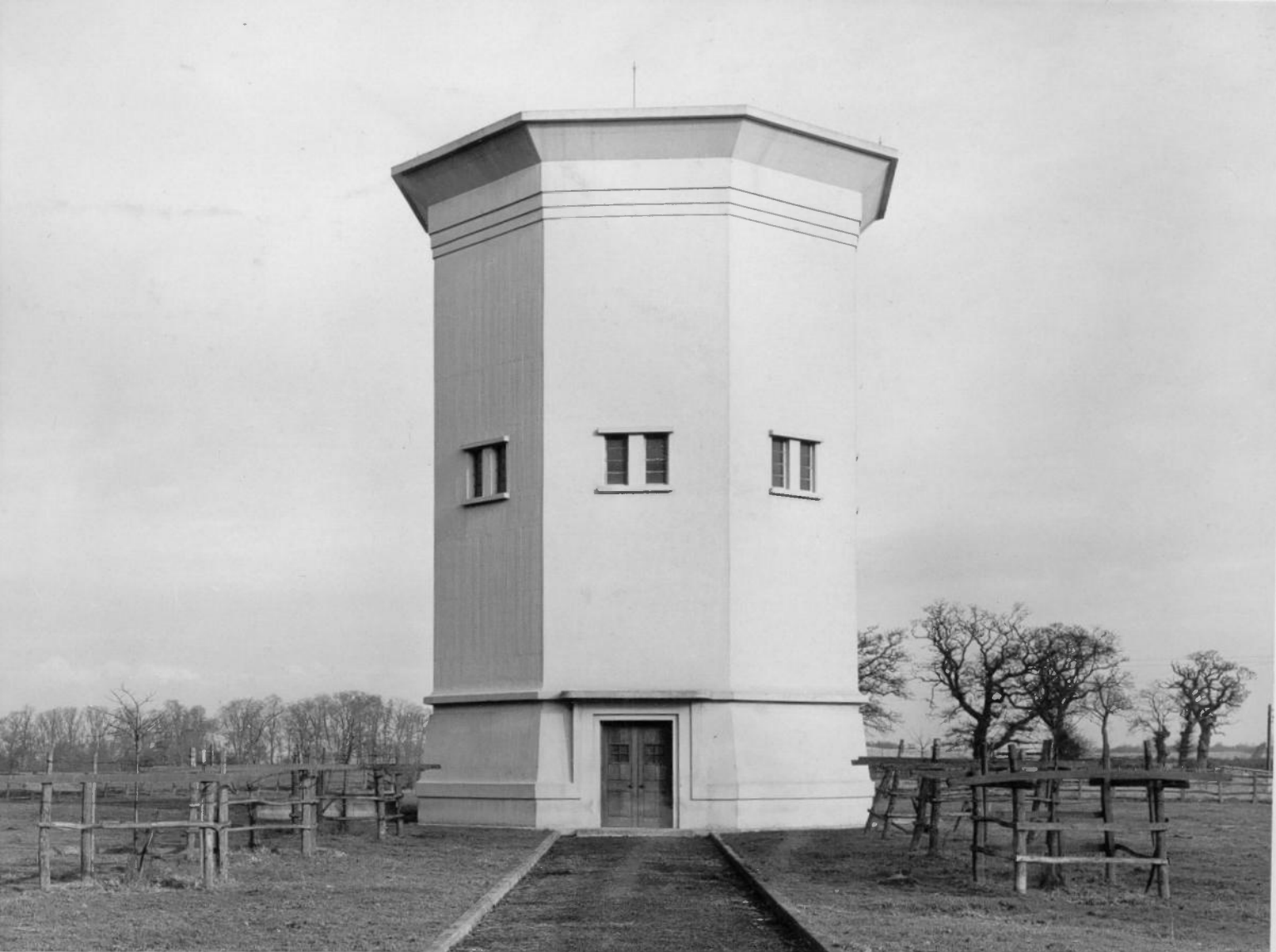
Rockingham Water Tower 17th January 1950
