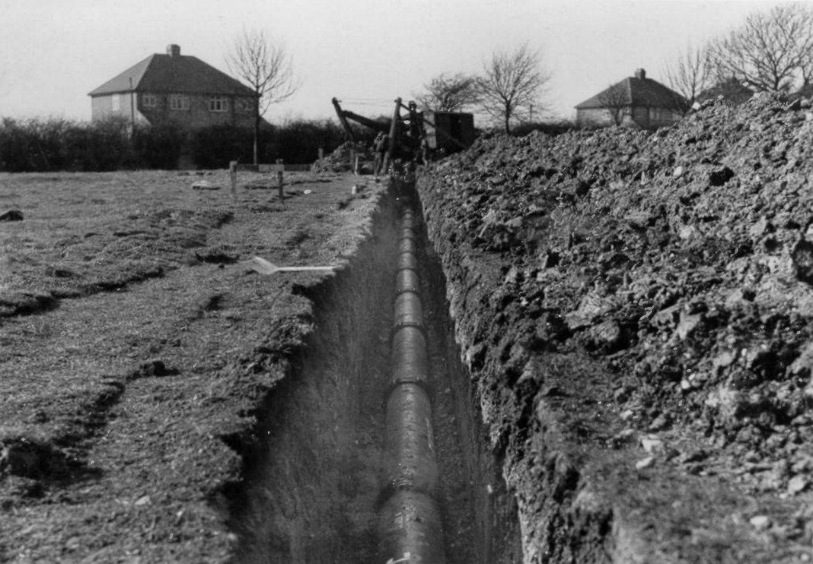
Corby pipe line 1943 (Everite 14")
