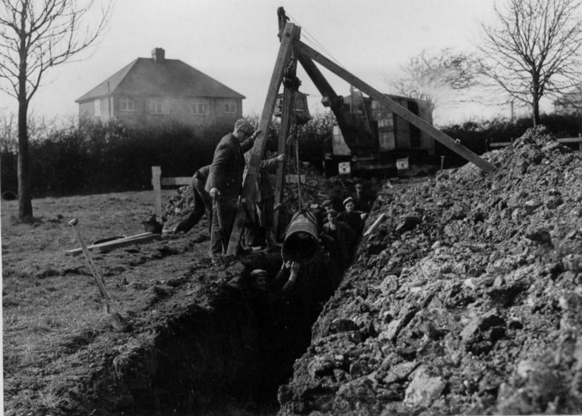
Corby pipe line 1943 (Everite 14")
